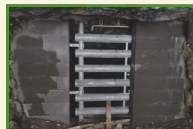
New closure of Velké Prepadlé adit
