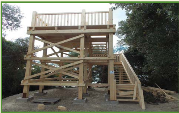
Observation tower at Hrušovská zdrž reservoir
