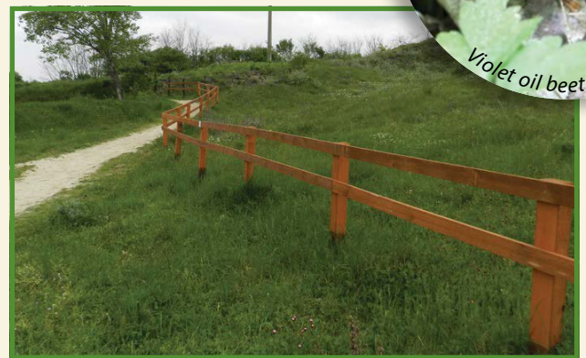
Restoration of fencing at Sandberg site at Devínska Kobyla
